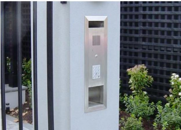
*Custom fabricated audio intercom and access control keypad panel in brushed stainless steel mounted into custom recessed housing (housing by builder).*
